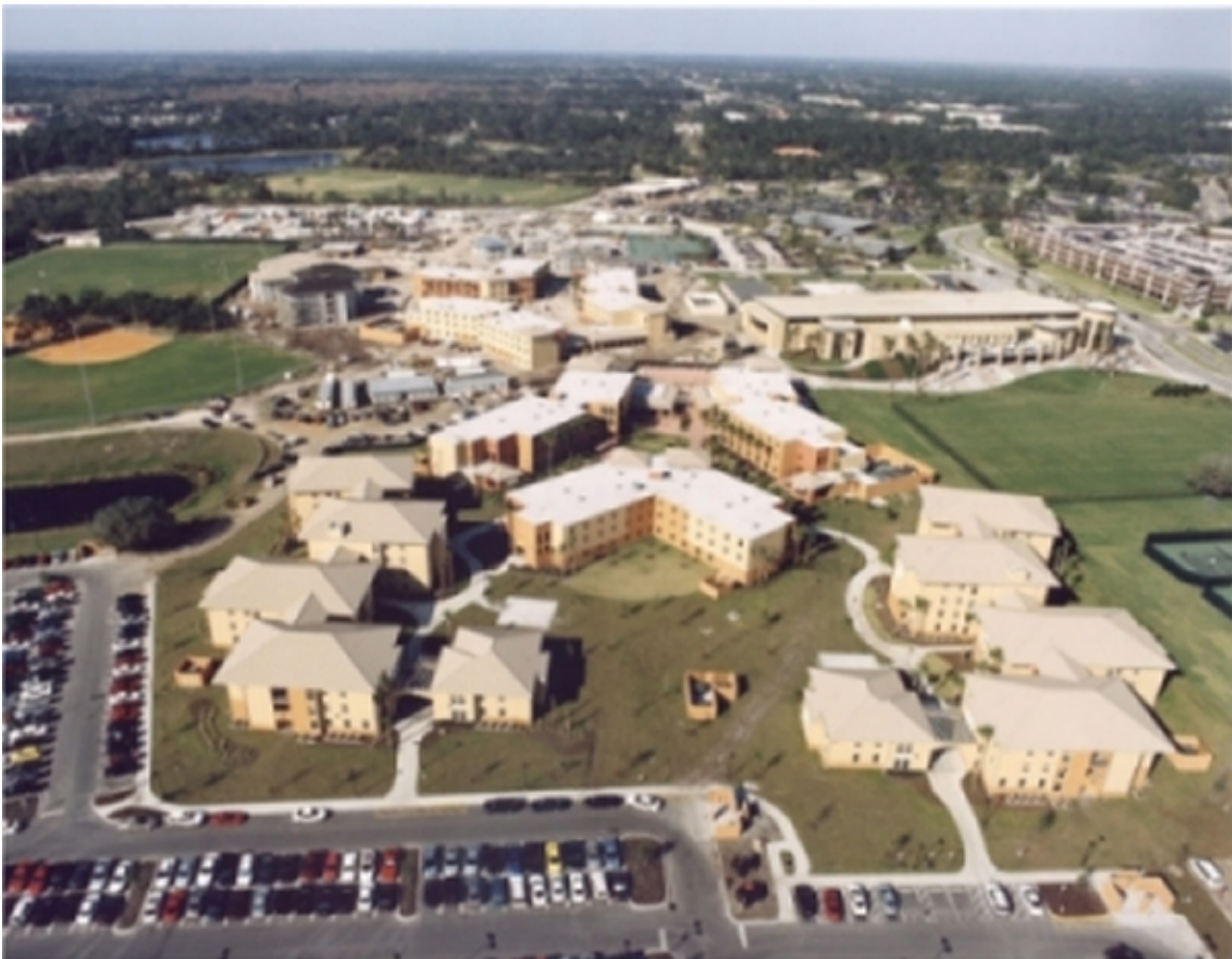
Figure 1: Sky view of Academic Village complex (Courtesy of Hanbury Evans Wright Vlattas & Co.)
